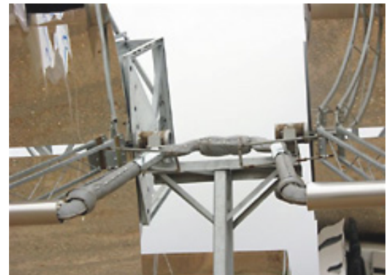
Double Solar Ball Joints
